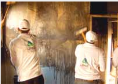
During: Volunteers from Jawwal cleaning the cinder on the walls of the home
