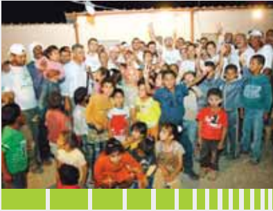
Volunteers from PG employees building two classrooms at Fasayel/Jordan Valley
